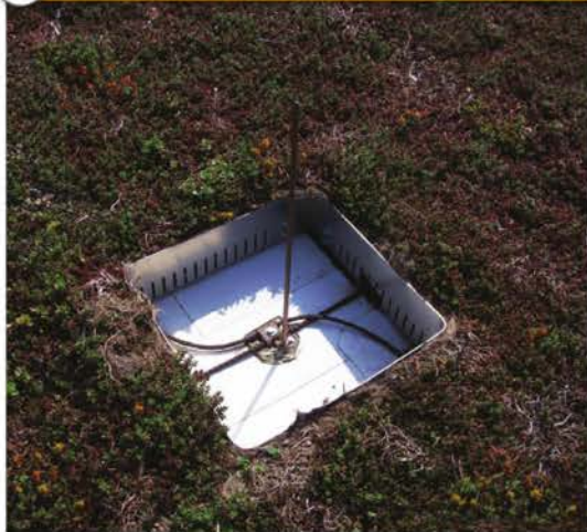
At the cargo facility (left), rooftop conductors are covered with soil and plants while air terminals are left exposed. An air traffic control facility (right) exceeded industry standards, ensuring operational security even during worst-case scenarios. For this project, rooftop conductors were elevated above the plantings on stanchions and extra-long air terminals were specified in order to simplify inspection.
