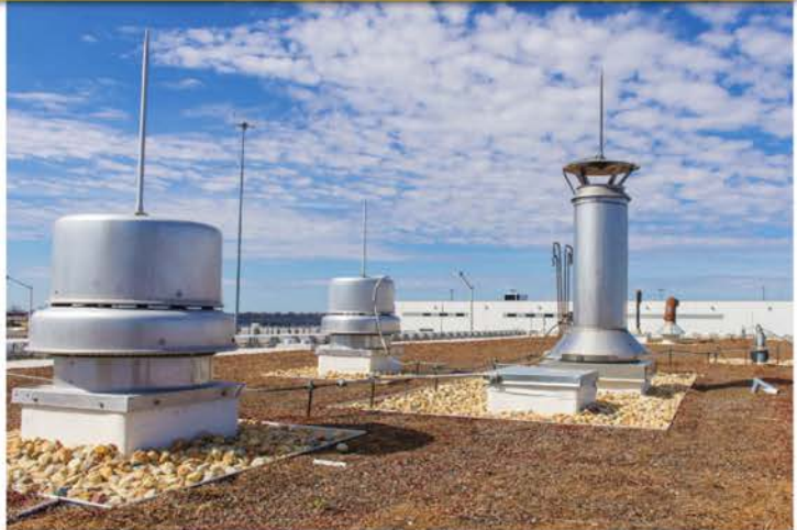
At the cargo facility (left), rooftop conductors are covered with soil and plants while air terminals are left exposed. An air traffic control facility (right) exceeded industry standards, ensuring operational security even during worst-case scenarios. For this project, rooftop conductors were elevated above the plantings on stanchions and extra-long air terminals were specified in order to simplify inspection.
